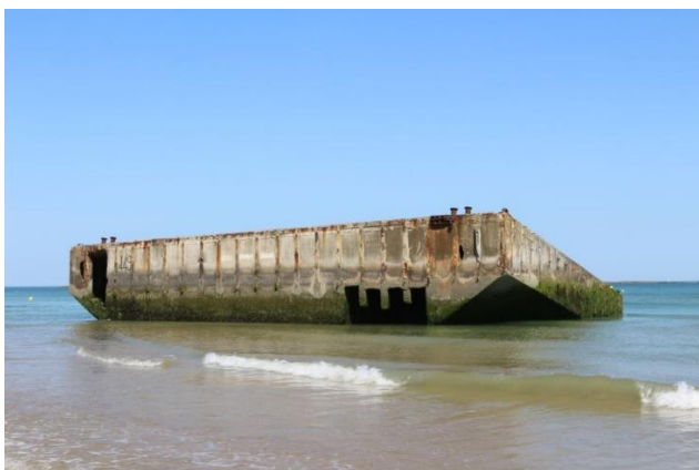
Remains of Mulberry Harbour at Arromanche. These artificial harbours were floated over the channel and used to enable cargo and men to be rapidly offloaded despite the shallow water of the beaches.
